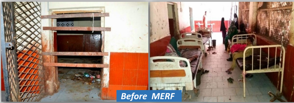
Accident & Emergency Unit (A&E) THQ Sujawal
