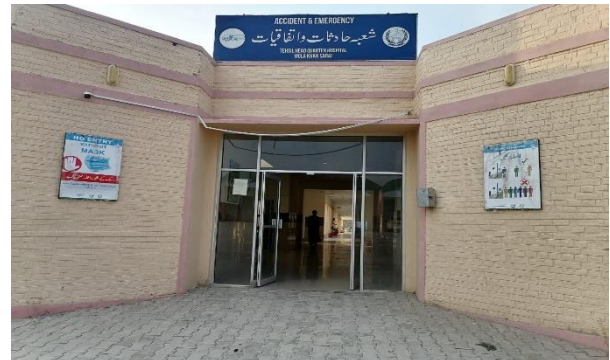
Accidental & Emergency Dept – Cat D Hospital Mola Khan Sarai
